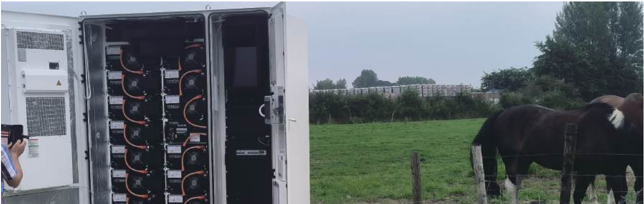
• The Netherlands 100kW/215kWh DH200F PV consumption (self-use)
